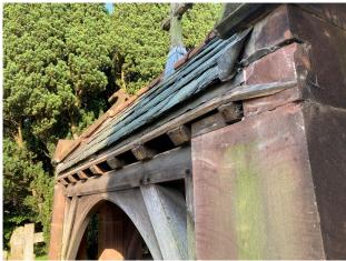
Rainwater in particular has rotted part of the oak boarding on that side of the roof where there does not appear to have ever been any guttering – unlike the south roof.
