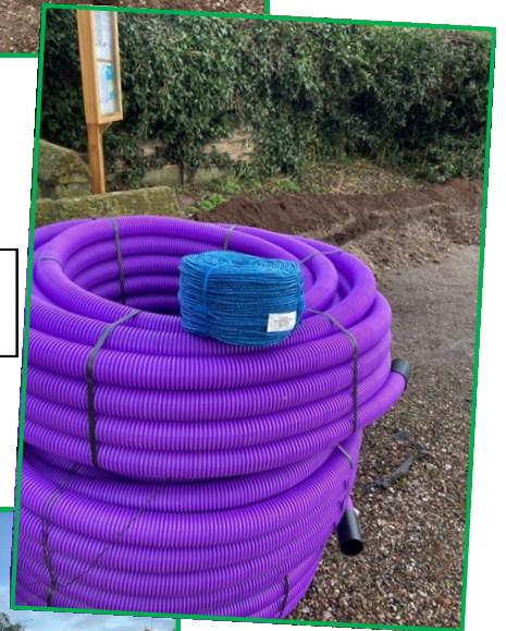
Ducting and draw rope
