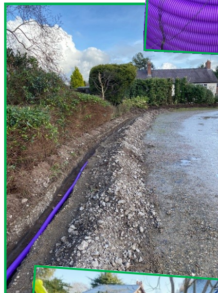
The trench in the car park
